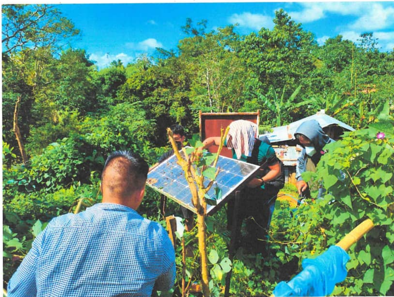
Cleaning the Solar Panels
